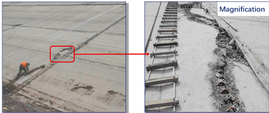
Fig. 1. Extrusion damage of face slab in post-earthquake Zipingpu CFRD.
